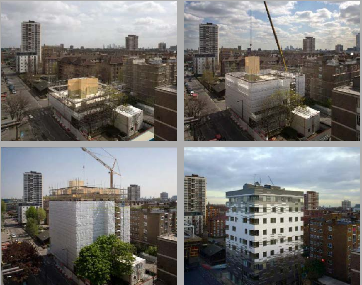
The Stadthaus, the first high-density housing building to be built from pre-fabricated cross-laminated timber panels
